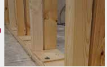
Separated stud - continuous sill and top beam
