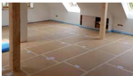
Loft conversion - PhoneStar installation in one layer
