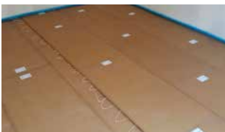
Modular construction - PhoneStar installation in multiple glued layers
